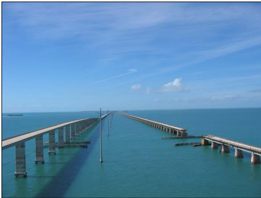
Looking south to KEYS' Service Area, high above the 7-Mile Bridge.
