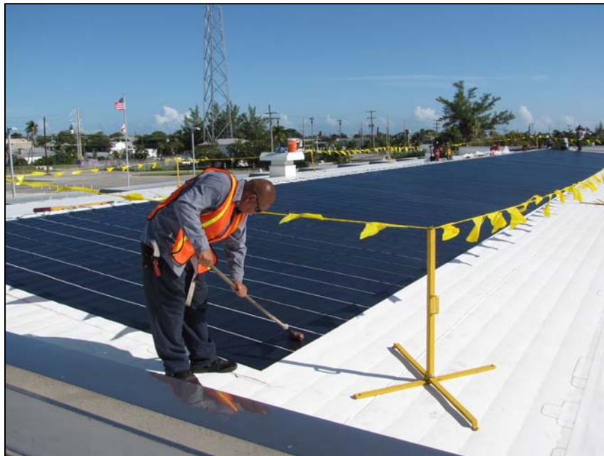
Installation of Solar Demonstration Unit at the Florida Keys Eco-Discovery Center.
